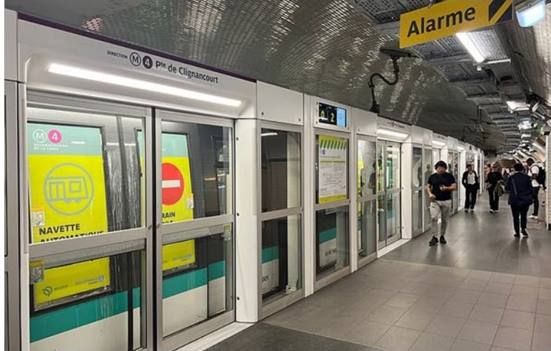
Paris Metro: Line 4 Platform Screen Door Testing
