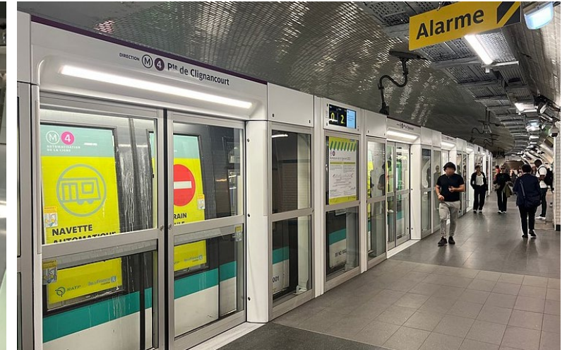
Paris Metro: Line 4 Platform Screen Door Testing
